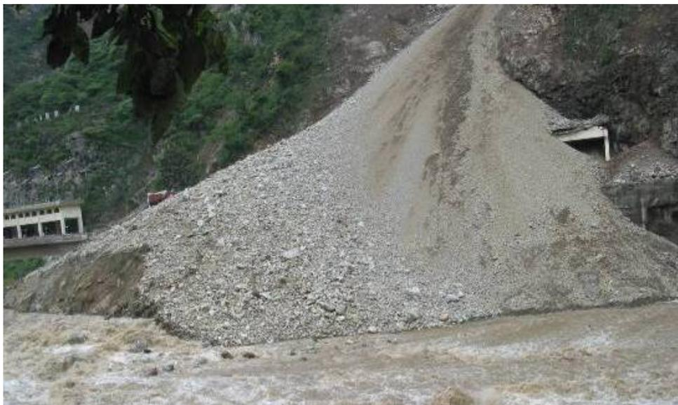
Figure 2: Tailrace of hydropower plant covered by landslide during the 2008 Wenchuan earthquake in Sichuan Province, China
