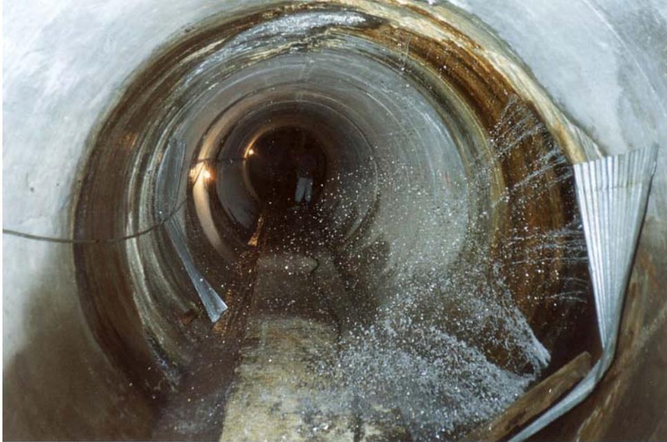
Figure 3: Leakage of existing fissure in bottom gallery of Sefid Rud buttress dam in Iran after the 1990 Manjil earthquake
