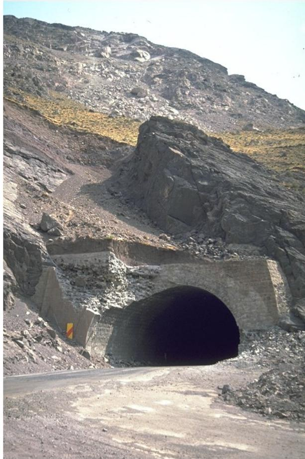
Figure 4: Tunnel portal damaged by rockfall during the 1990 Manjil earthquake
