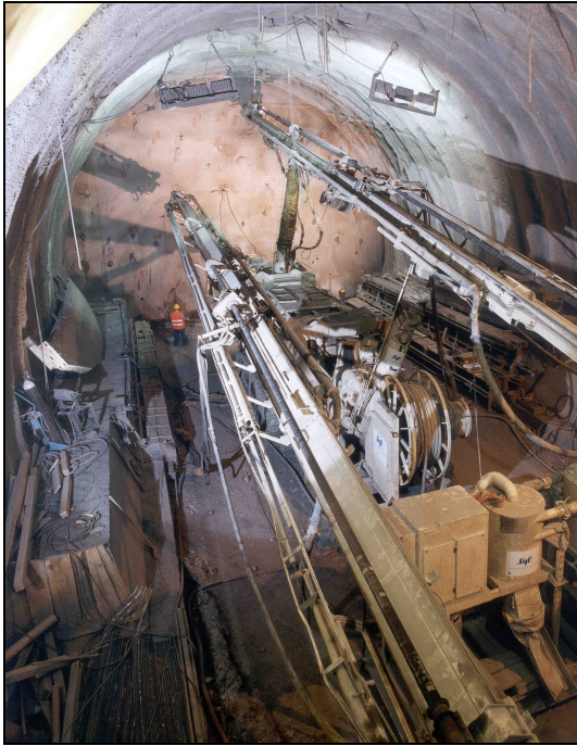
Figure 3 Full face excavation/construction method: face reinforcement and ring closure operations.
