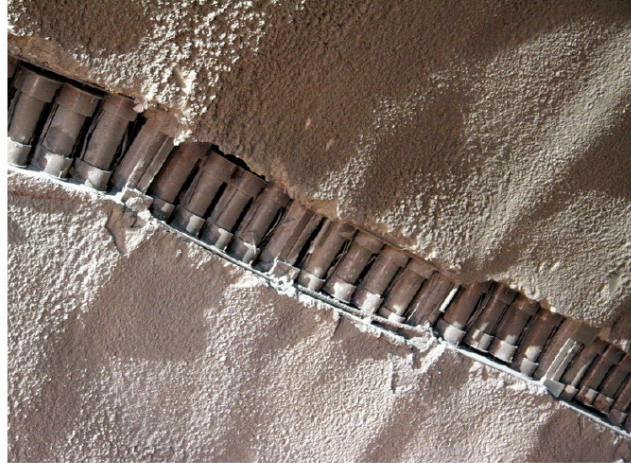
Figure 6 Yielding support with LSC elements incorporated in the shotcrete lining and between steel sets with yielding couplings [12].
