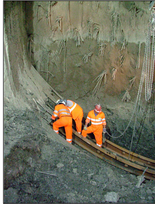
Figure 3 Full face excavation/construction method: face reinforcement and ring closure operations.
