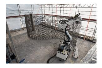
The In situ Fabricator building the Mesh Mould on Empa NEST. The Mesh Mould process unifies the reinforcement and formwork production into a single and robotically controlled on-site fabrication system.
