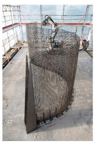
The In situ Fabricator building the Mesh Mould on Empa NEST. The Mesh Mould process unifies the reinforcement and formwork production into a single and robotically controlled on-site fabrication system.
