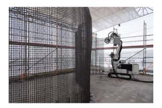
The concrete will be poured in once the mesh fabrication is completed. Activating the mesh as reinforcement renders it as a functional stay-in-place formwork, making the process inherently waste free.
