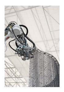
Close-up image of the fabrication process. The Mesh Mould toolhead bends and welds a 6 mm steel rebar to fabricate the mesh structure.
