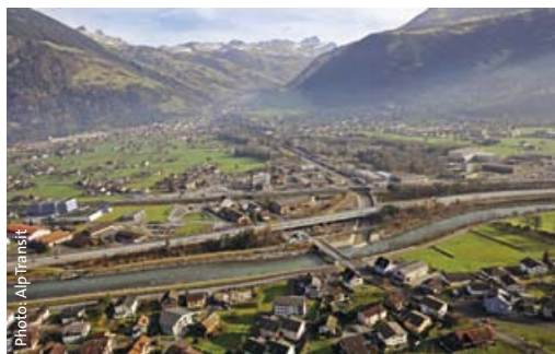
Photo: AlpTransit Lower Reuss Valley: a NEAT point of entry and a test planning area.
