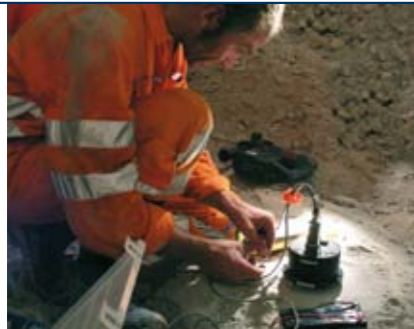
The SED is installing a seismometer in the Gotthard Base Tunnel.
